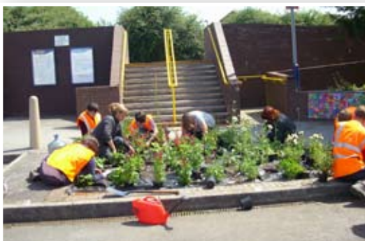
Planting the new garden at Weston Milton
